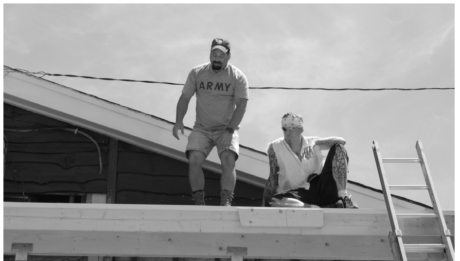
Above: Chico DeGrace (l) and Duane Houghton working on the new awning roof, Memorial Day weekend.
