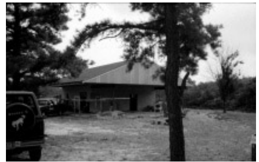
The 1989-2005 Trading Post, construction nearly complete. (Photo courtesy Tom Bednarz).
