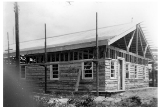
Siding work on the "admin" side of the 1966-1987 Trading Post (Photo courtesy Dennis Prefontaine).
