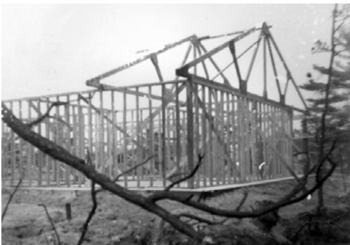
Construction begins on the 1966-1987 Trading Post. (Photo courtesy Dennis Prefontaine)
