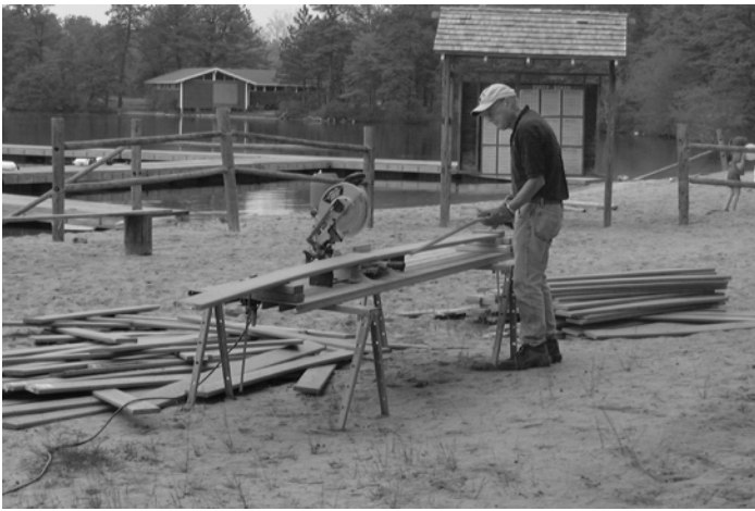
Alum Al Stiles cutting decking to size to be installed on the waterfront docks, Memorial Day Weekend 2006
