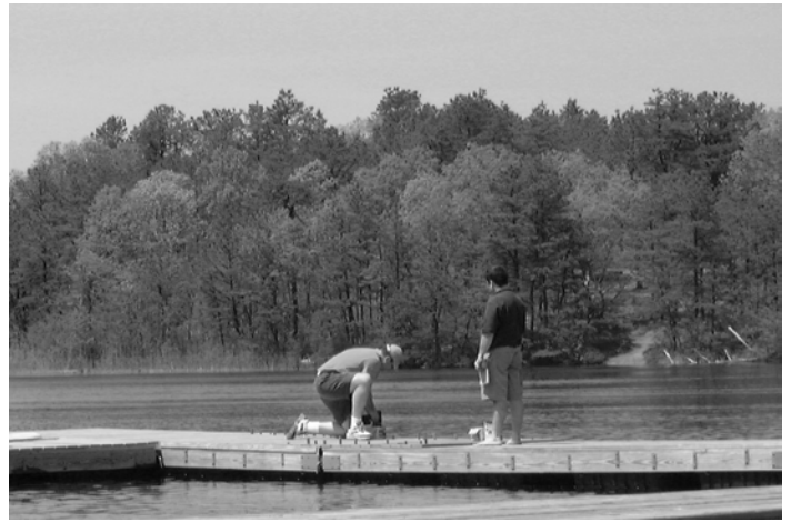
Alums screwing down the new decking on the waterfront docks, Memorial Day Weekend 2006
